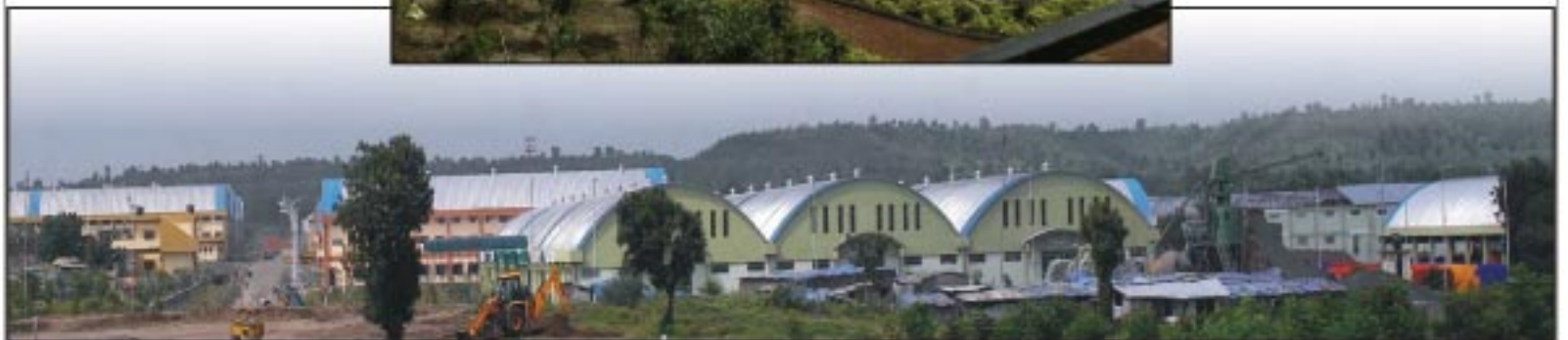
A mega project at Gadegaon
